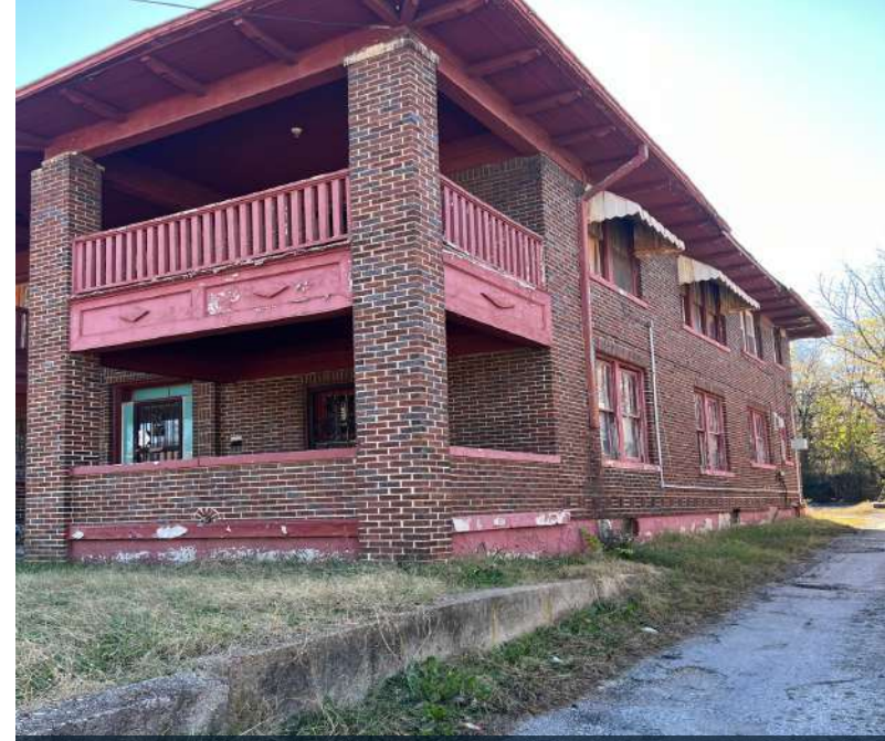
Along the right side of the property, there is an asphalt driveway to the rear.
