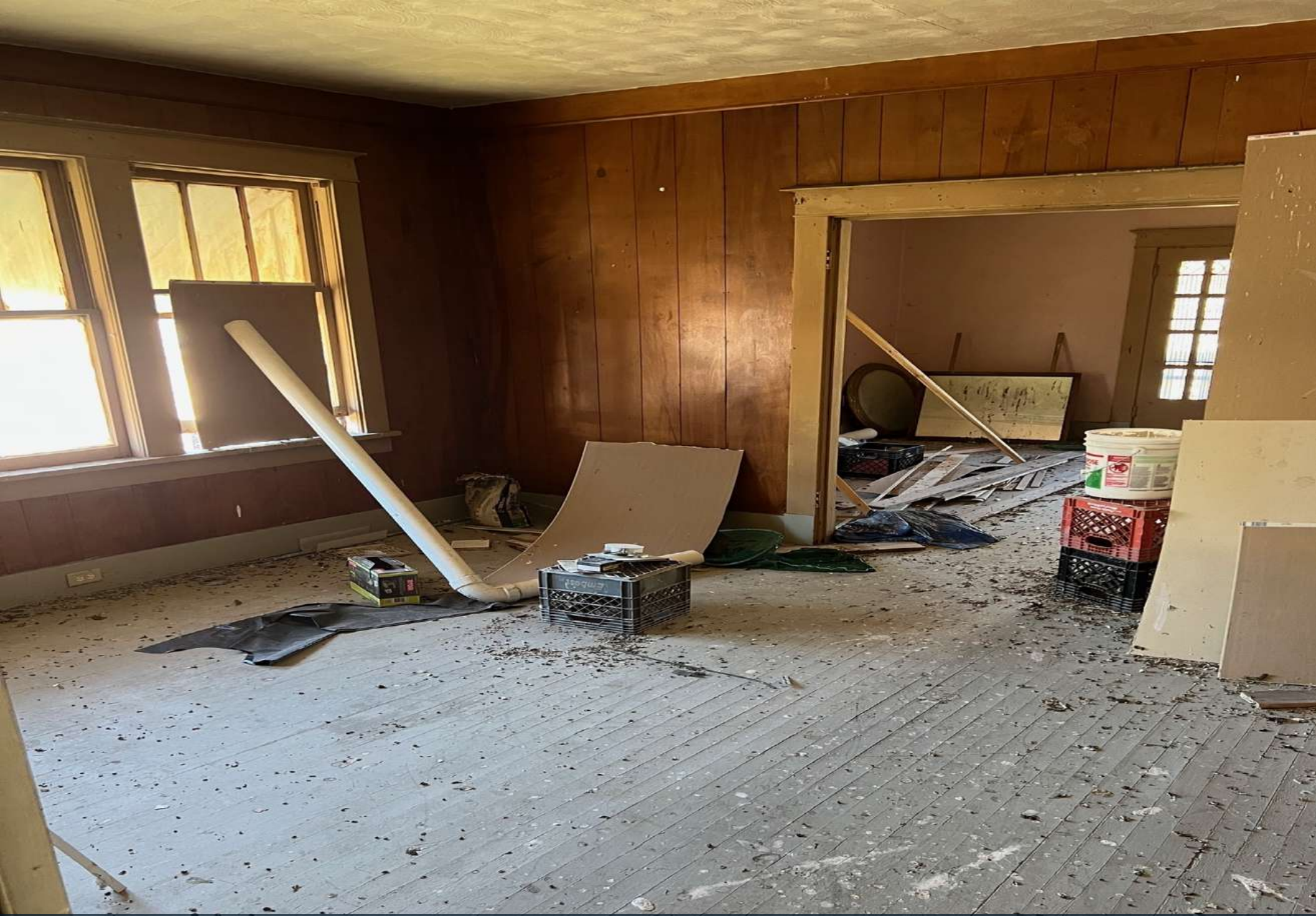
The living room is in the middle of both bedrooms and has the interior entrance to the unit.
